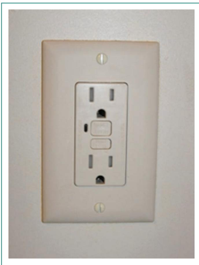
**Figure 10.23** A GFCI With Three-Pronged Receptacle
