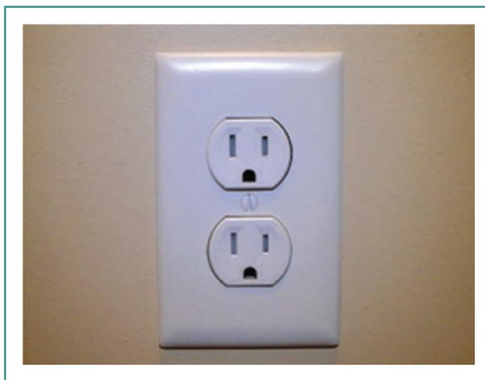
**Figure 10.21** A Polarized Receptacle
